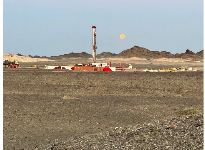
Pilot well drilling at Nomgon
