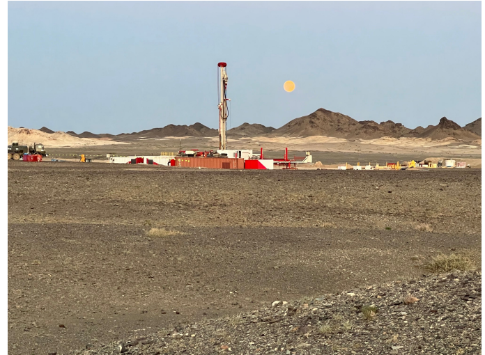
Pilot well drilling at Nomgon
