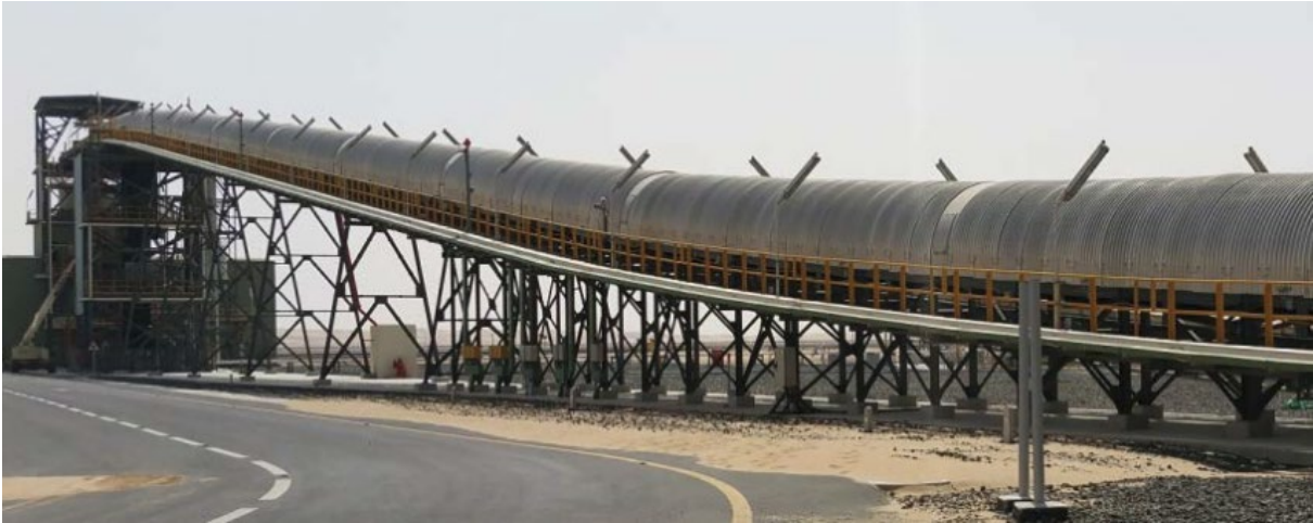
Photo 2: Reference Belt Conveyor and Transfer Tower
