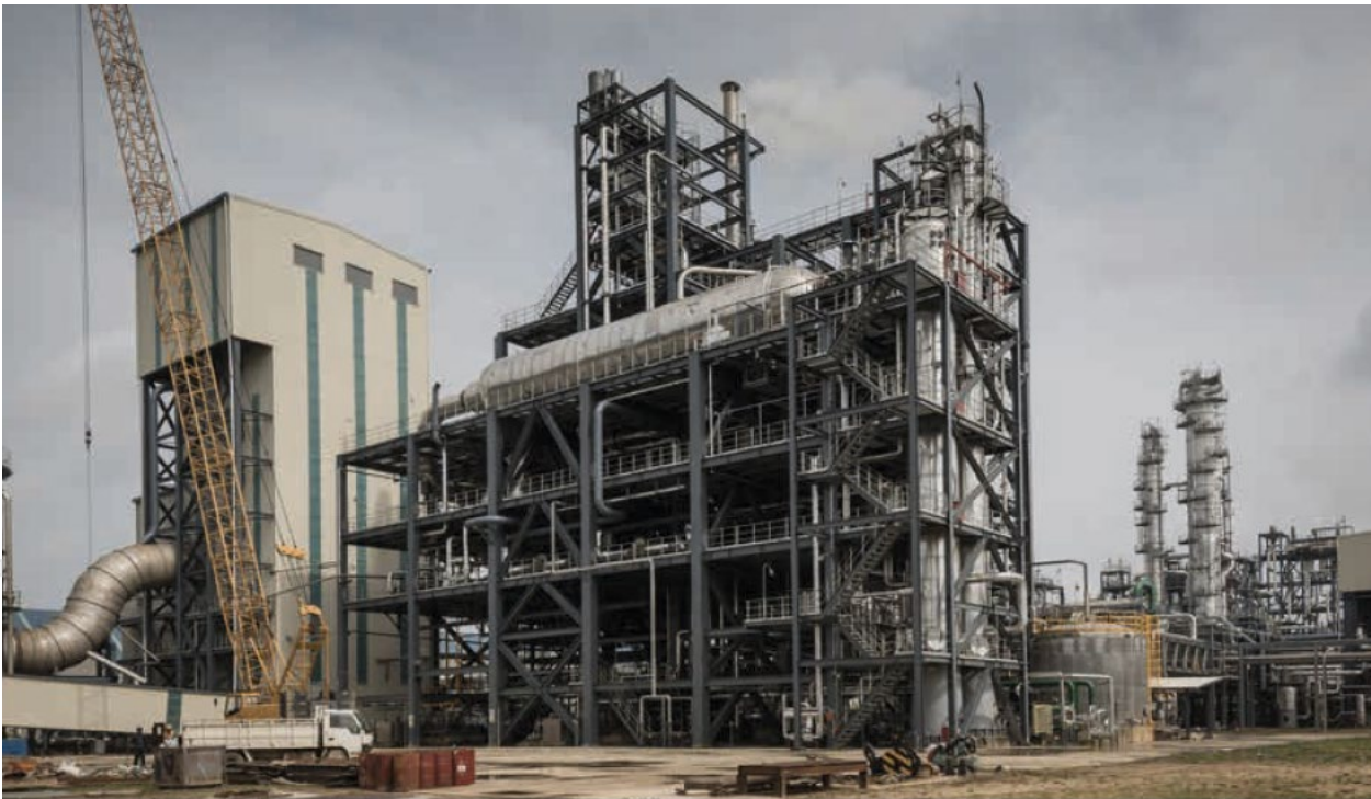
Photo 1: Typical Stamicarbon Urea Plant reactor
