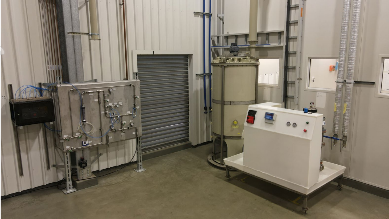
Figure: Control and safety systems being installed and commissioned
