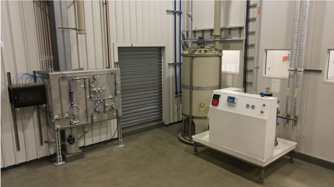
Figure: Control and safety systems being installed and commissioned
