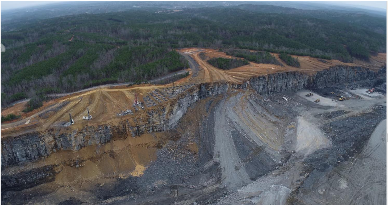
Image: Black Warrior Mine: new drills on top bench; D11T dozer push paths; benching to Newcastle seam; then to Mary Lee seam
