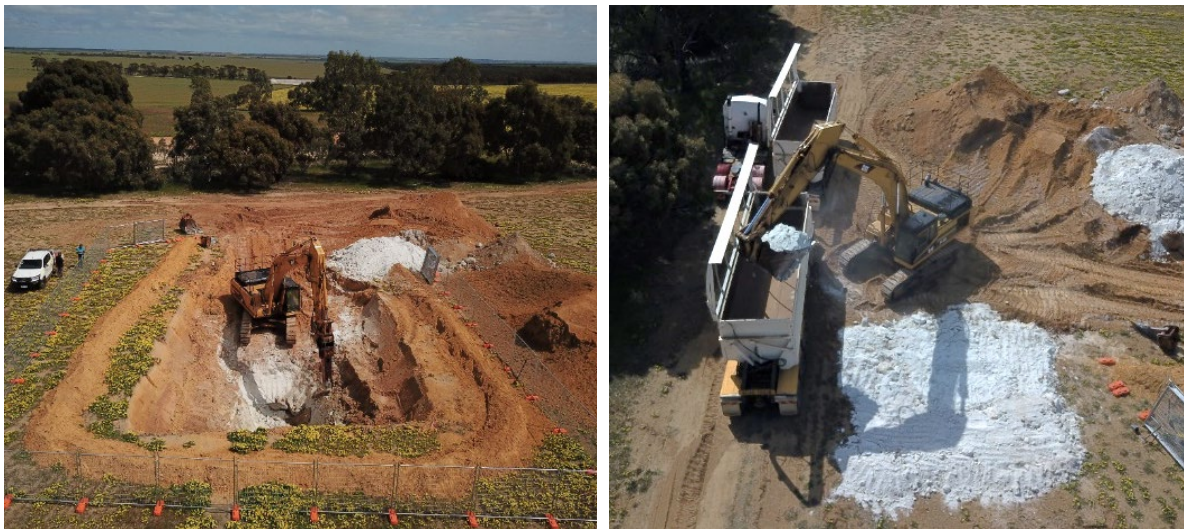
Figure 8: Test-pit in progress
