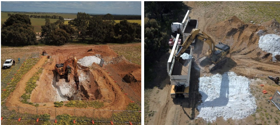
Figure 8: Test-pit in progress
