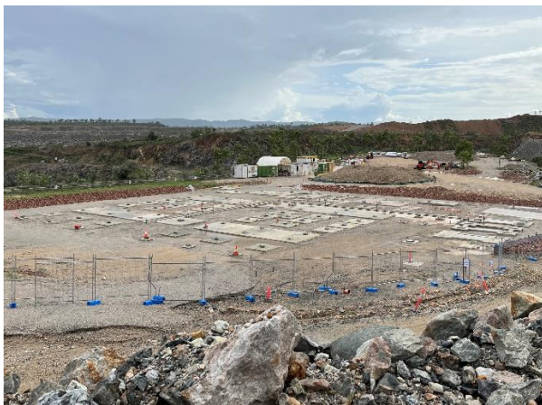
Figure 3: K2 Hydro substation foundations completed - 19 December 2022
