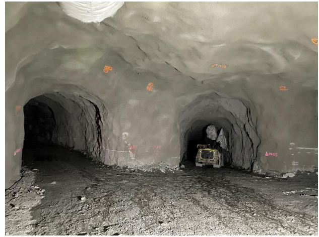
Figure 2: MAT, new Y-Junction completed - 14 December 2022
