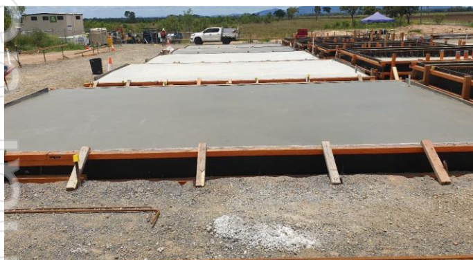
Figure 7: Megapack foundations
