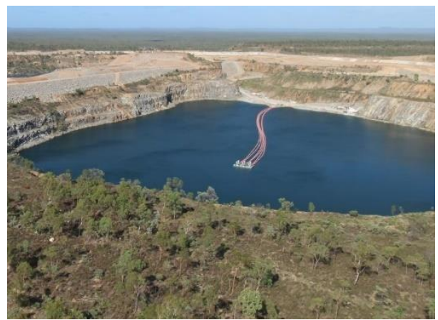
Figure 4: Dewatering pontoon and pipeline in Eldridge Pit - 21 December 2022
