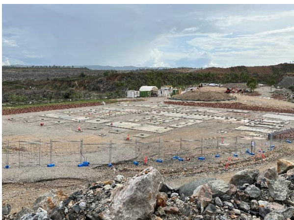
Figure 3: K2 Hydro substation foundations completed - 19 December 2022
