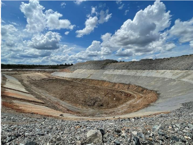
Figure 1: Intake Canal, cement stabilised crusher dust placement - 18 December 2022
