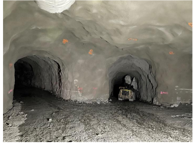
Figure 2: MAT, new Y-Junction completed - 14 December 2022
