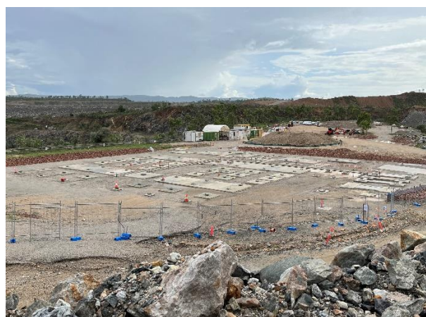
Figure 3: K2 Hydro substation foundations completed – 19 December 2022
