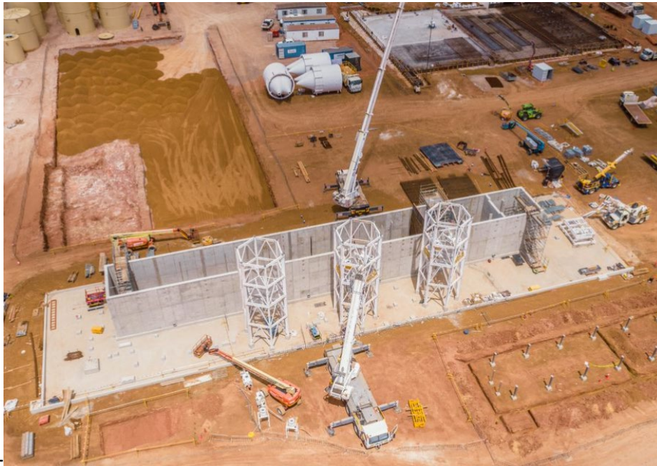
MgO Tanks. Outer walls complete, two inner walls completed, silo structures installed. Excavation for load in system and Chemicals warehouse in the rear.
