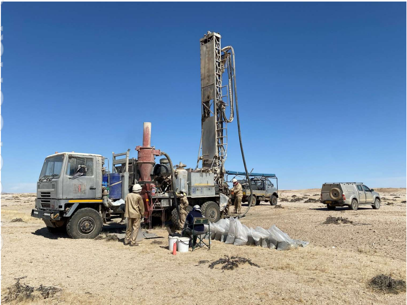
Figure 2 Drilling at Koppies 4
