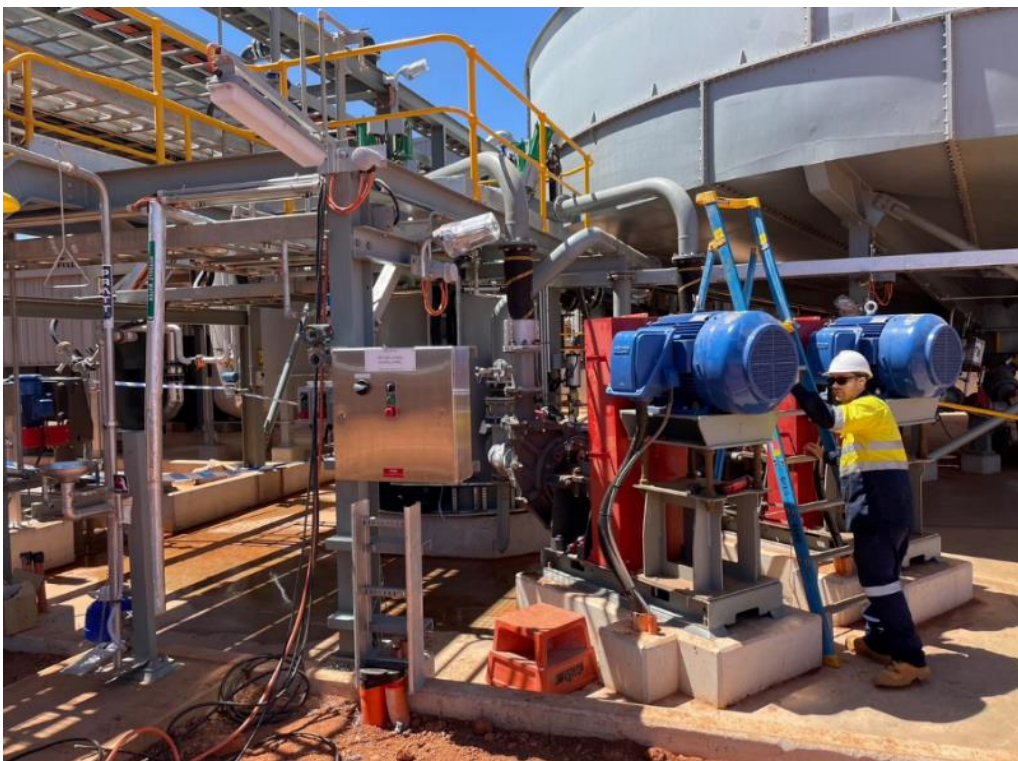
Figure 13 – Tails concentrate thickener pumps commissioning (December 2022).
