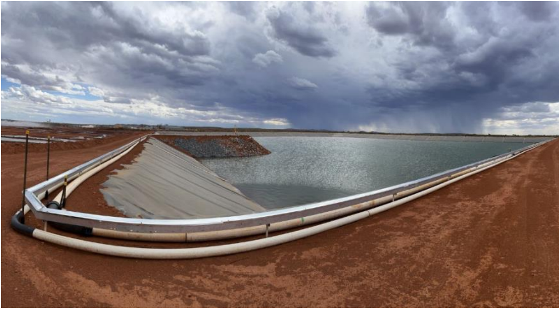
Figure 14 – Tailings storage facility TSF (December 2022).
