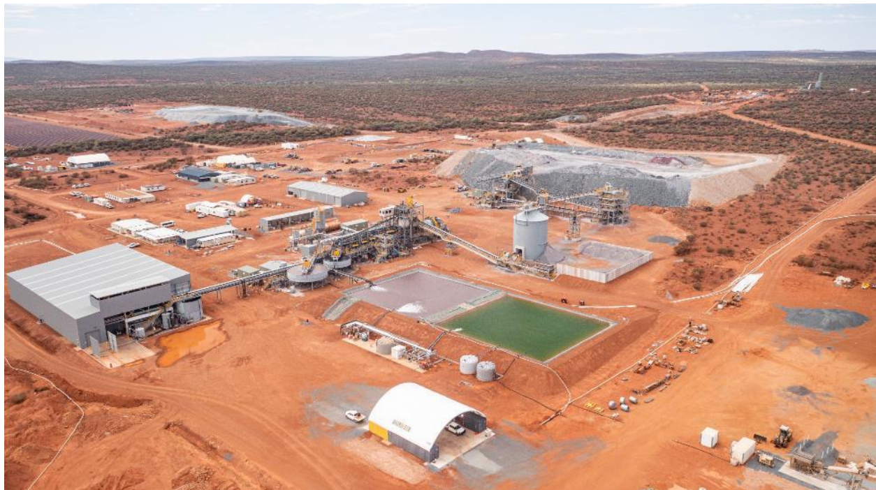
Figure 3 – Abra processing plant and mine site commissioning January 2023 (Photo – 20 January 2023).
