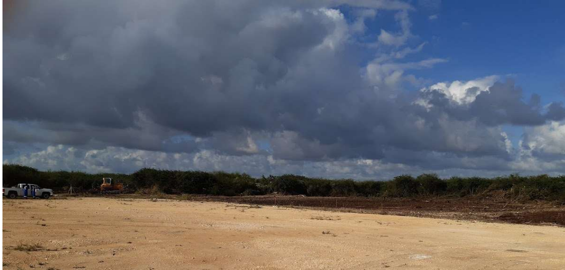
Figure 2 – Alameda pad expanded to accommodate production storage tanks
