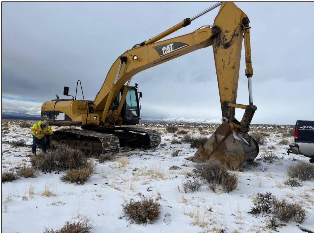
Image 2 – Clearing the drill pad after recent heavy snow at the Nevada Lithium Project (illustrating that the Project is accessible all year round)
