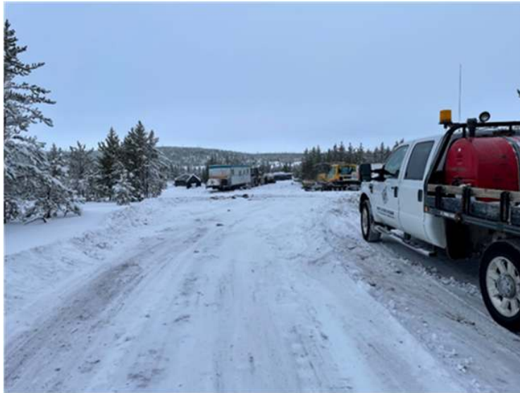
Figure 4 – New Pasfield Lake Base Camp under construction in January 2023.
