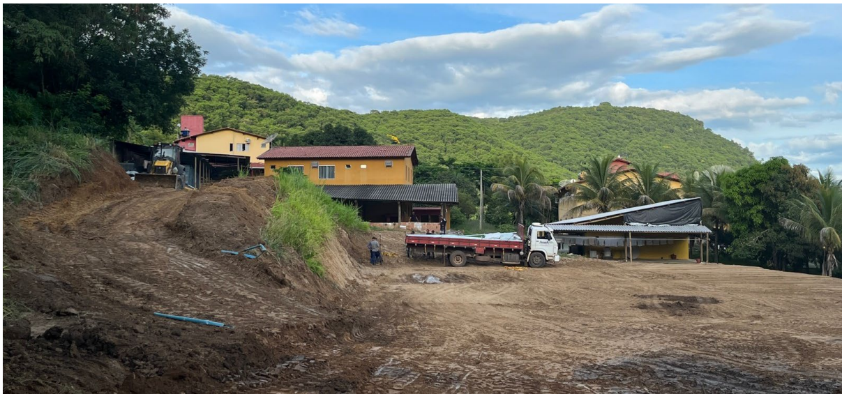
Figure 5: Site construction work underway in early January 2023, to expand the existing core processing and storage facility on site at the Salinas Project in Brazil
