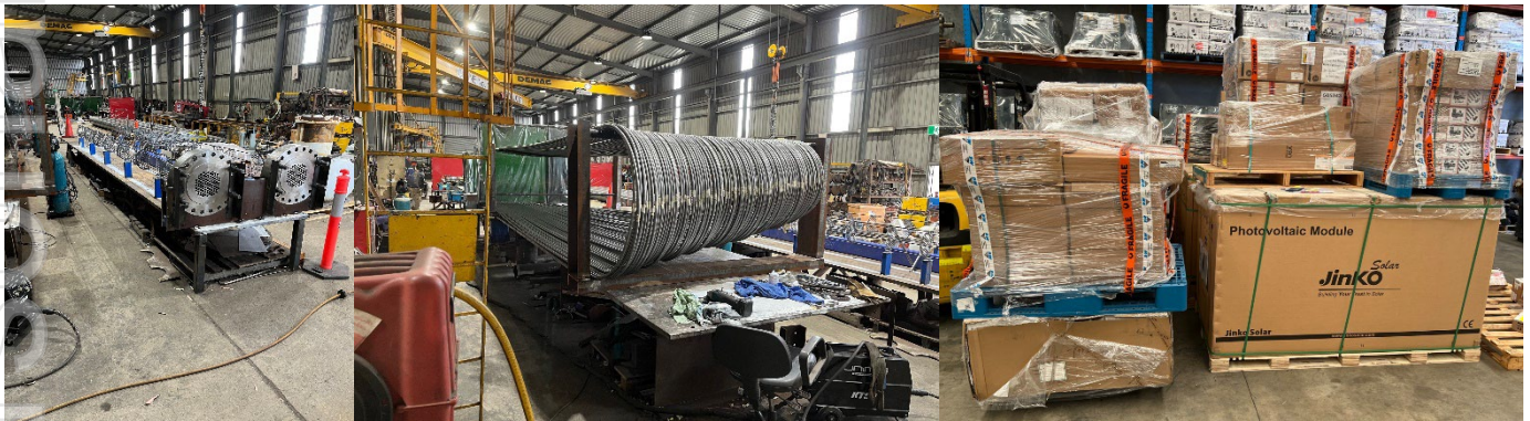
Above: Fabrication of Heat Exchanger for Walyering upstream facility and arrival of solar package to power the facility
