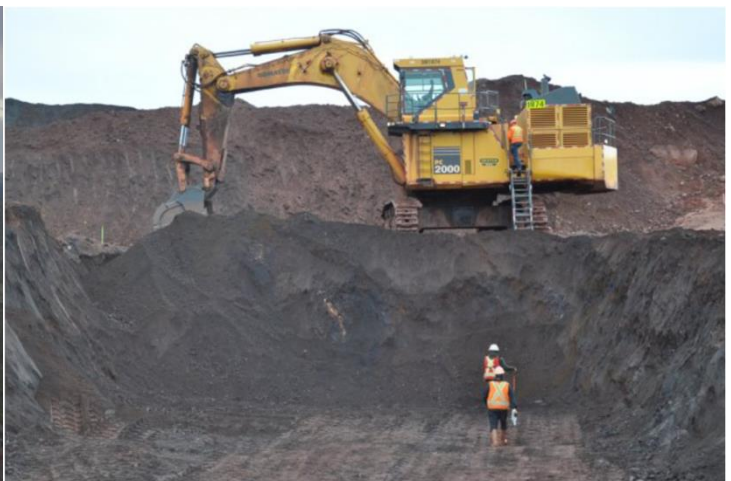
Figure 6: Previous Trenching Work 3
