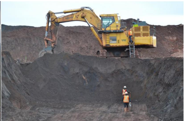
Figure 6: Previous Trenching Work 3
