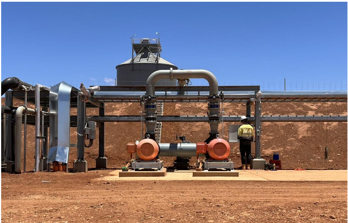
Figure 15 – Water services area pump installation.
