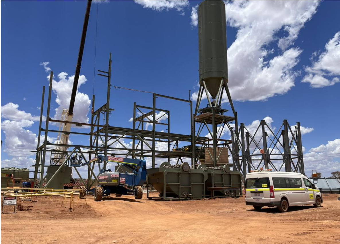
Figure 14 – Paste Plant Structural Steel being erected.
