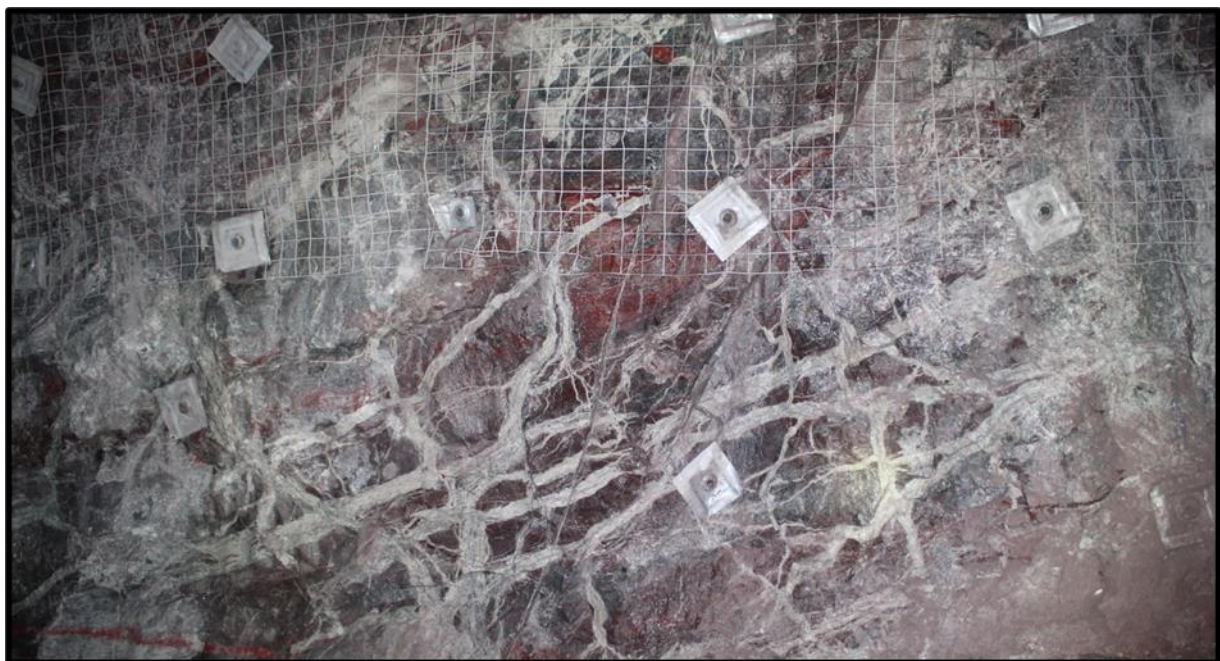
Figure 4 – Image of the ore face underground in 1300 mRL access drive showing various orientations of the barite/carbonate veins.
