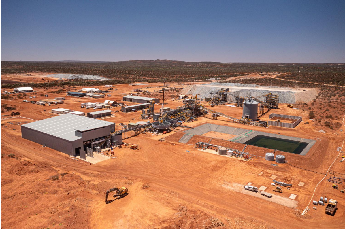
Figure 6 – Aerial photo of the Abra processing plant (Photo 18 November).
