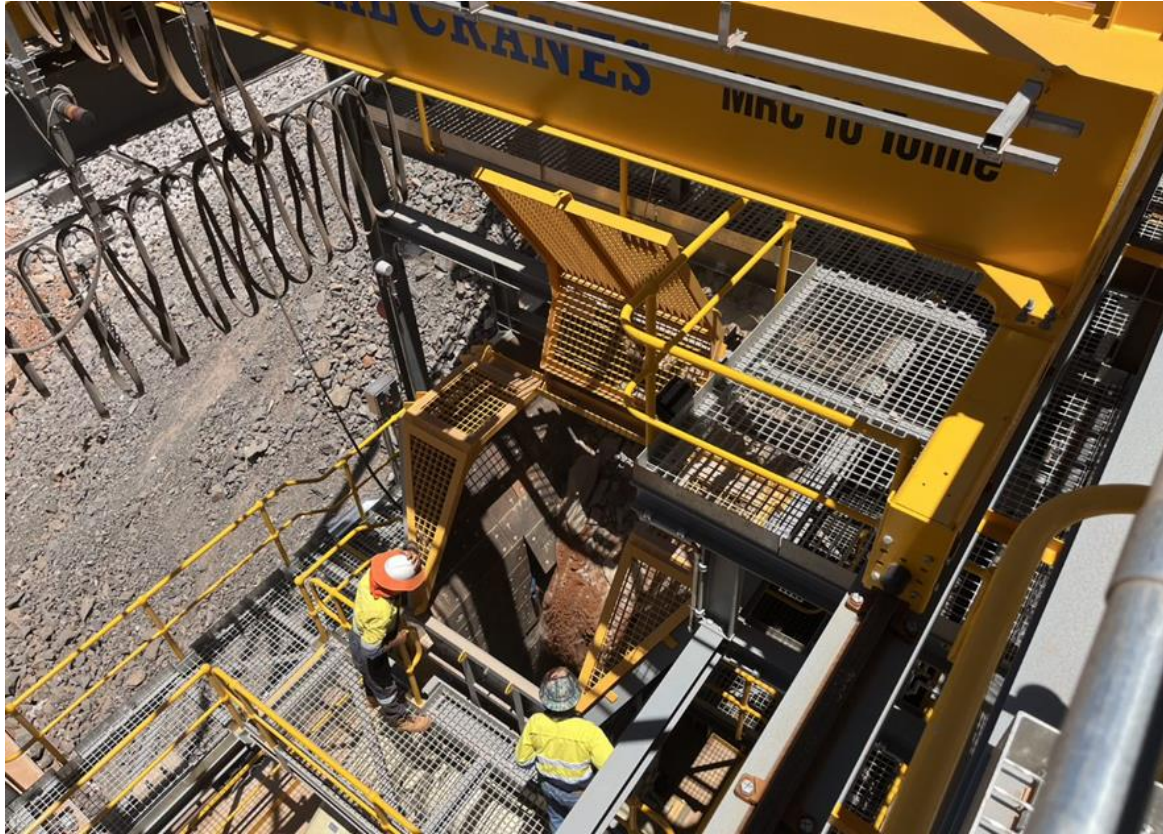
Figure 8 – Inspecting first material through the crusher.
