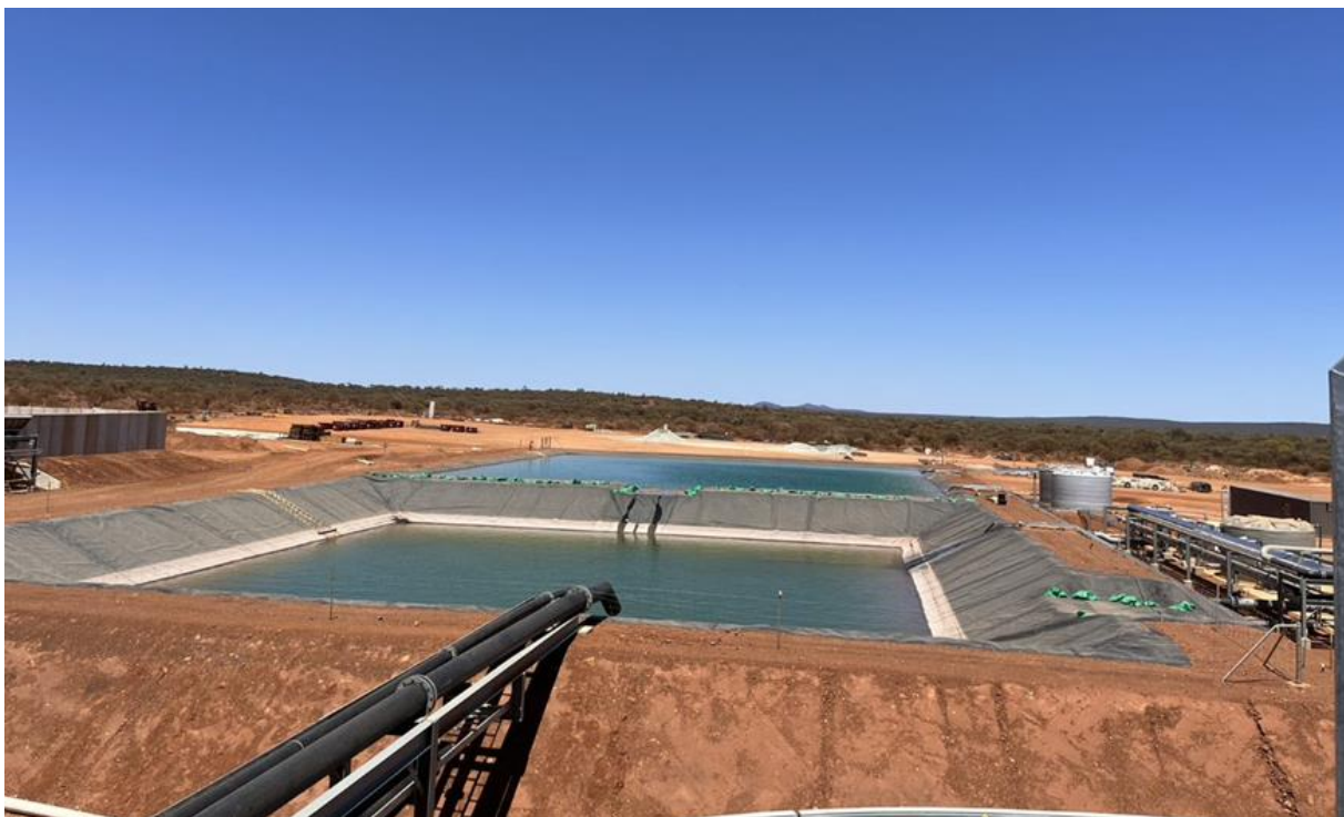
Figure 11 – Raw water and process water dams filling up.
