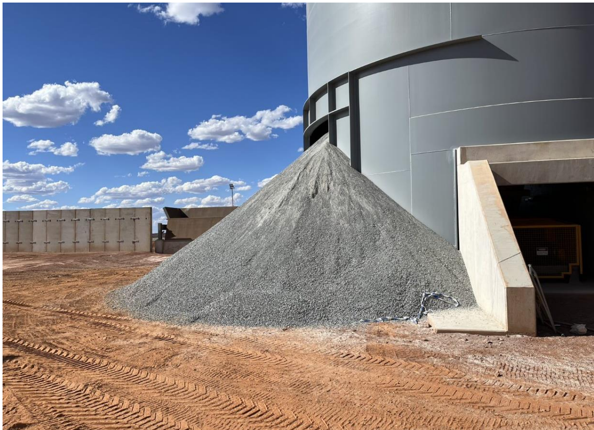
Figure 9 – Fine ore bin filled with inert waste.
