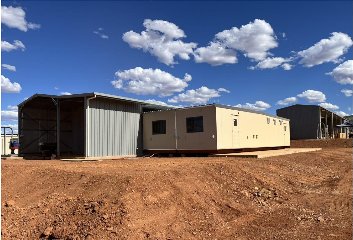
Figure 16 – Laboratory demountable buildings landed into position.
