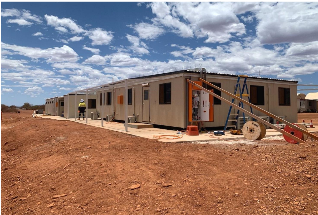
Figure 17 – Processing plant office buildings and changerooms.
