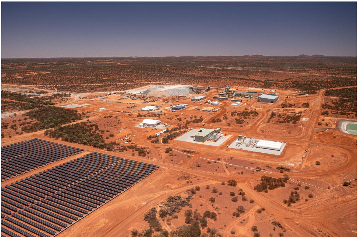
Figure 7 – Aerial photo of the Abra solar farm and power station with the Abra processing plant in the background (Photo 18 November).
