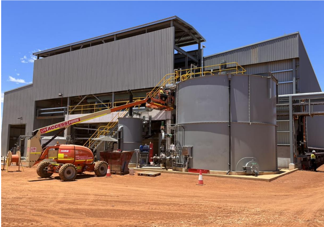
Figure 18 – Concentrate shed tank wiring installation.
