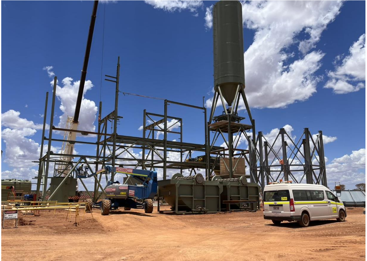
Figure 14 – Paste Plant Structural Steel being erected.
