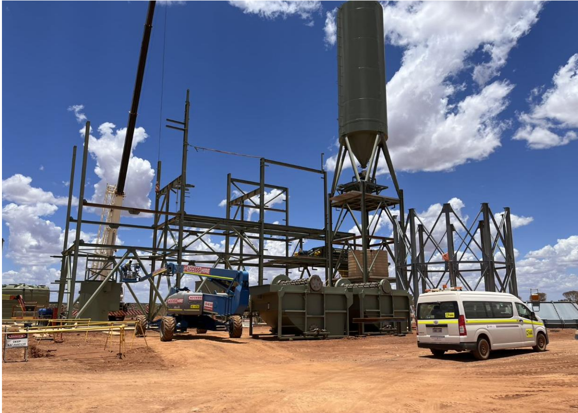
Figure 14 – Paste Plant Structural Steel being erected.
