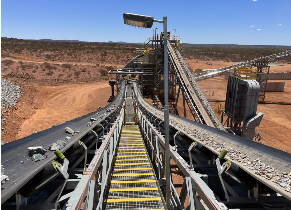
Figure 2 – Crushing and screening plant commissioning (Photo 26 November).
