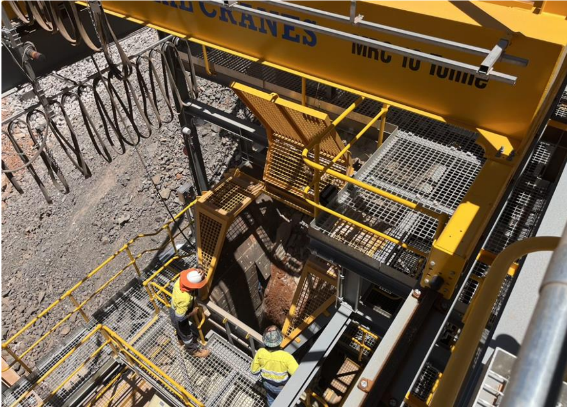
Figure 8 – Inspecting first material through the crusher.
