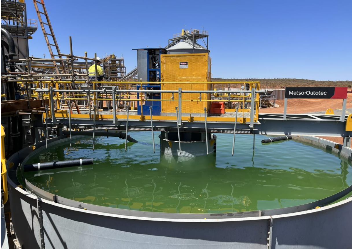
Figure 12 – Concentrate thickener full of water.
