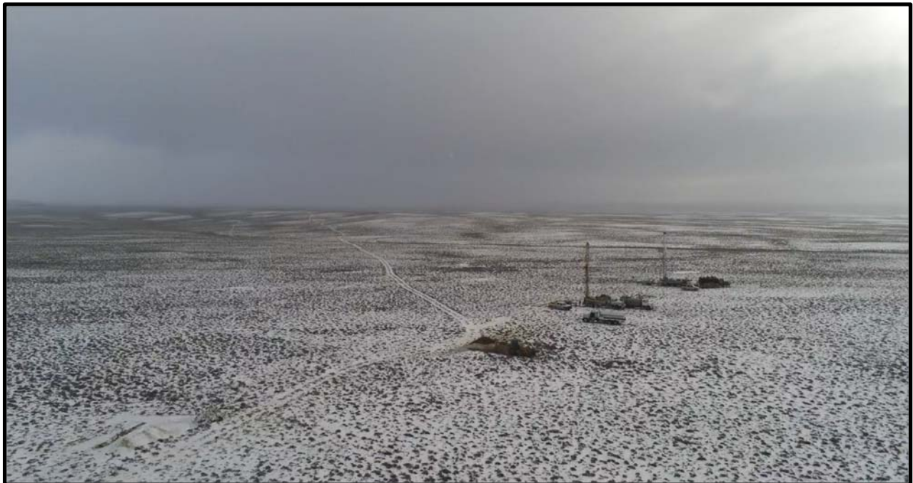
FIGURE 1. MUD ROTARY DRILL RIGS OPERATING, ODIN ISR URANIUM PROSPECT, GDB (WY).
