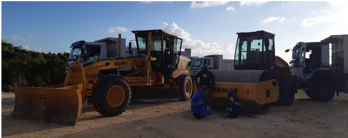
Figure 2 - Civil contractors arriving at the Alameda well pad to commence work
