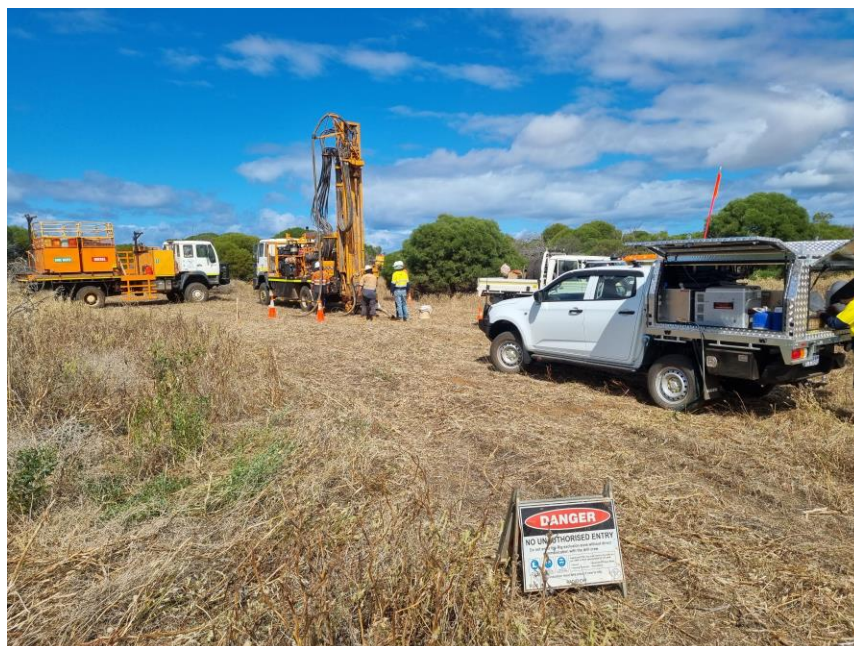
Figure 1: Bostech drilling rig at Port Gregory
