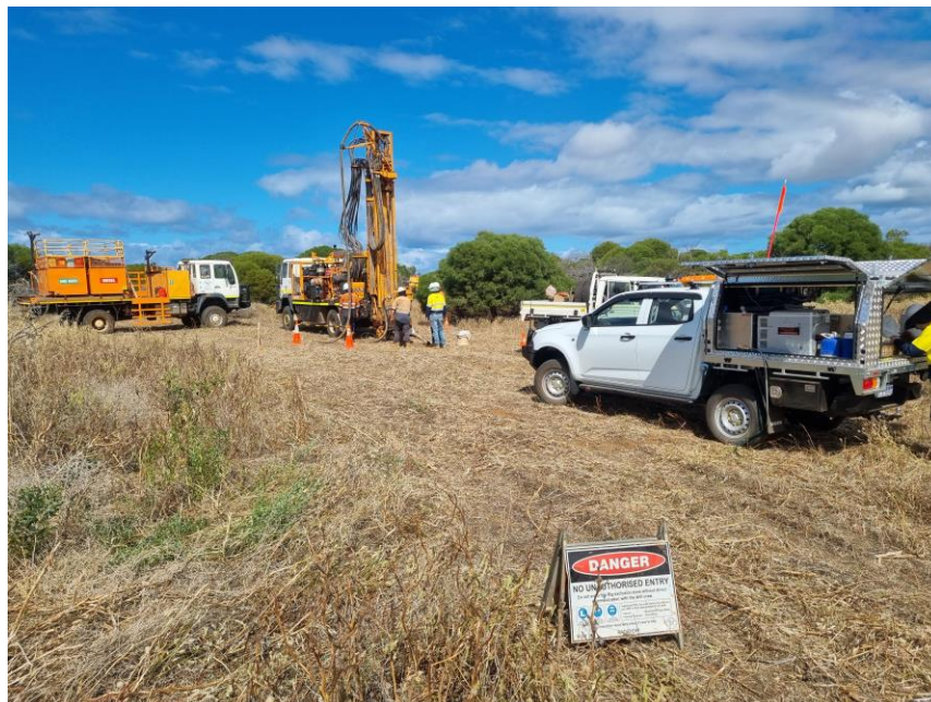
Figure 1: Bostech drilling rig at Port Gregory
