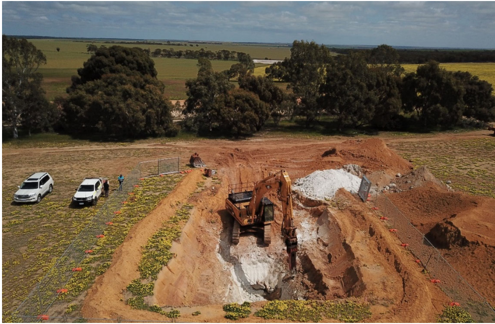
Figure 2: Bulk sample test pit showing thin colluvial cover and white kaolinitic saprolite clays
