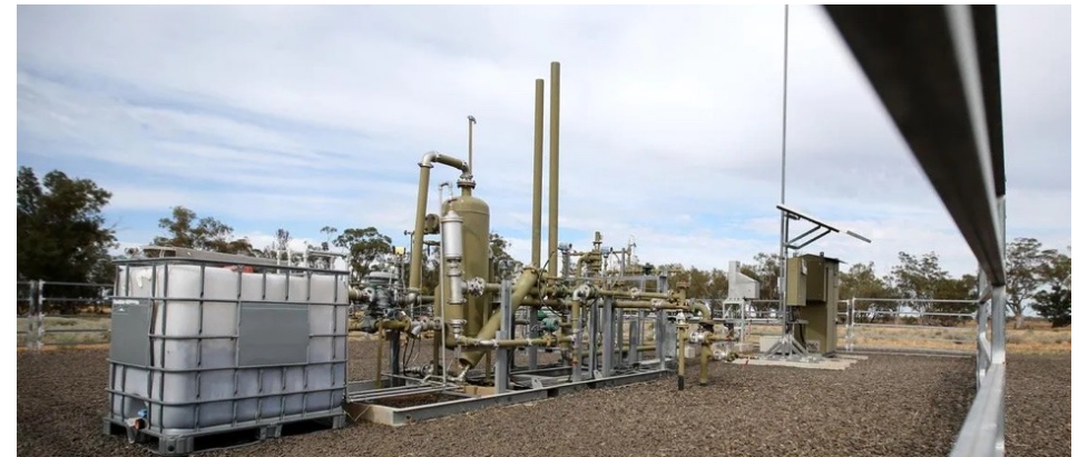
Santos – Narrabri CSG Project, in New South Wales, Australia.
