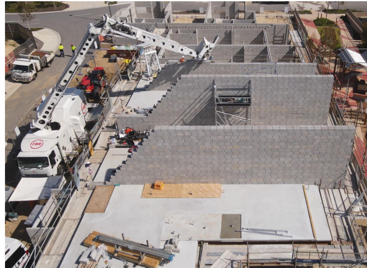
8 metre triple-leaf walls at 16 townhouse Willagee development
