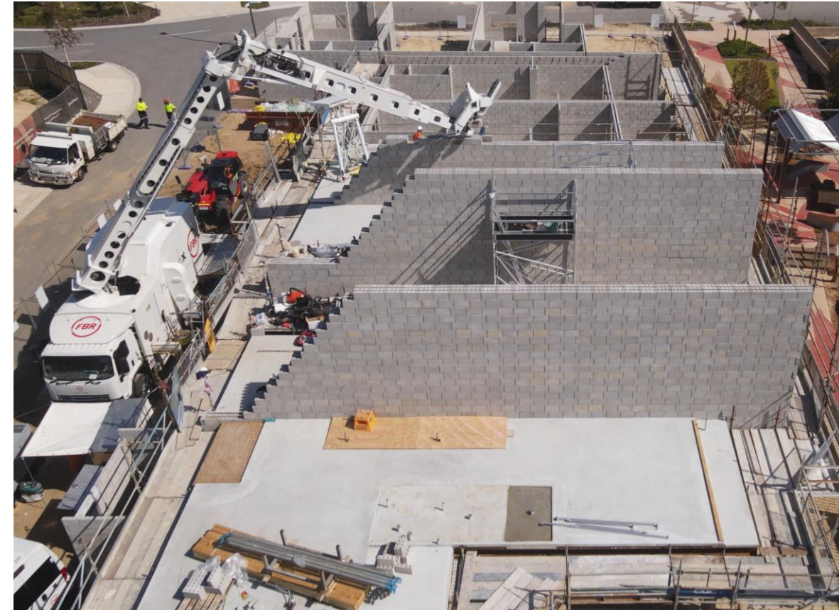
8 metre triple-leaf walls at 16 townhouse Willagee development
