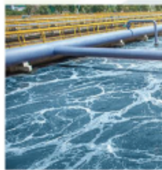
Wastewater treatment plant
