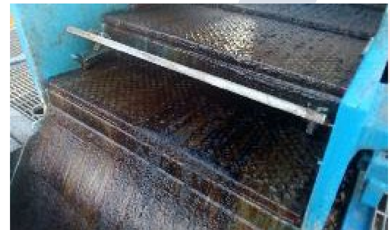
Oil on the shakers at Alameda - 1
