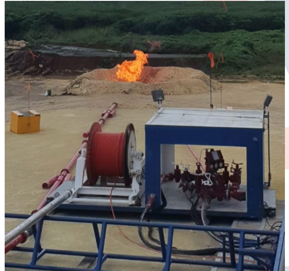
Flaring operations whilst drilling Alameda-1 - Block 9, Cuba
