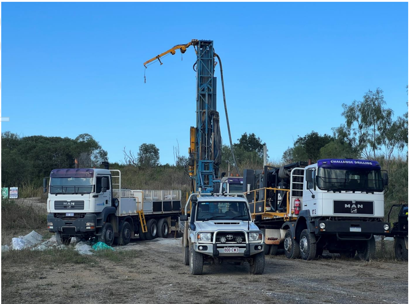
Figure 12: Drilling underway at QMines Mt Chalmers mine site, September 2022.
