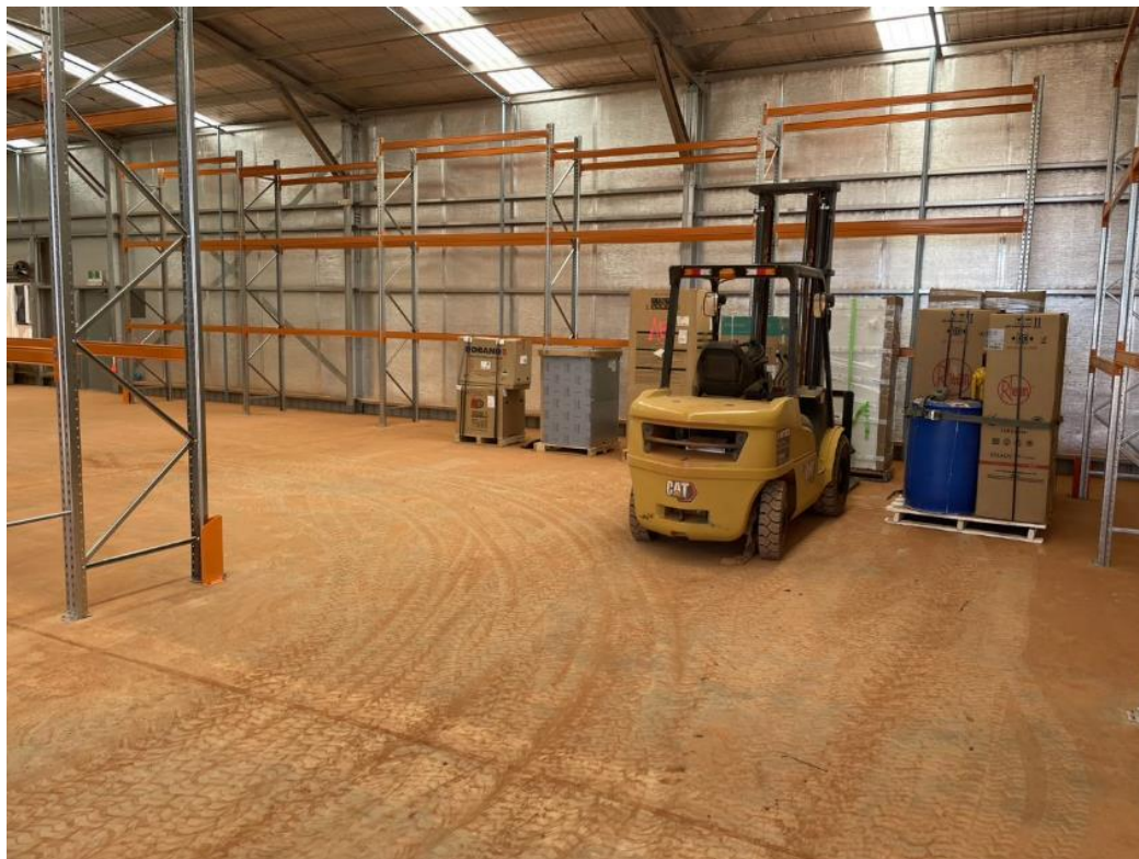
Figure 17 – Surface stores installation.
