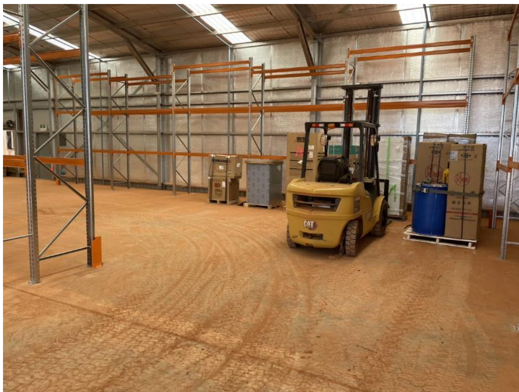
Figure 17 – Surface stores installation.
