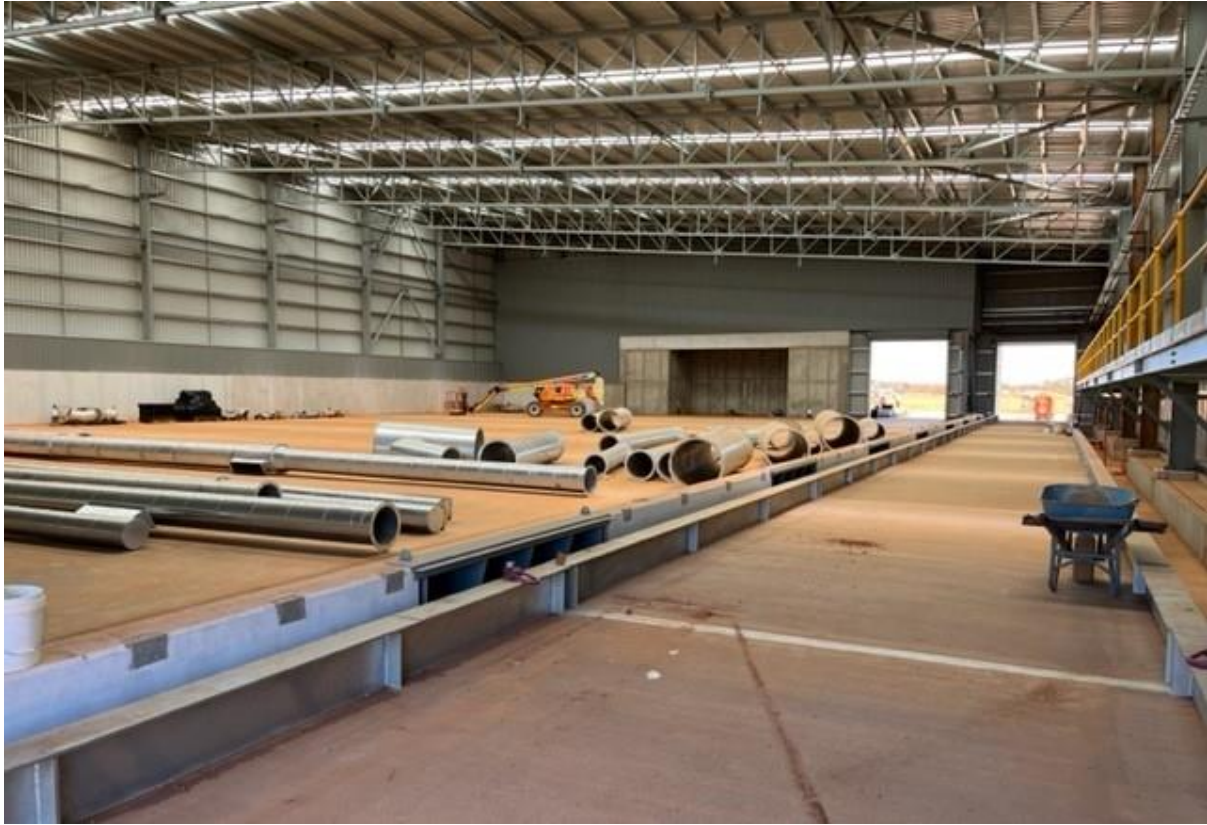
Figure 11 – Inside of concentrate storage shed (Photo 11 November).
