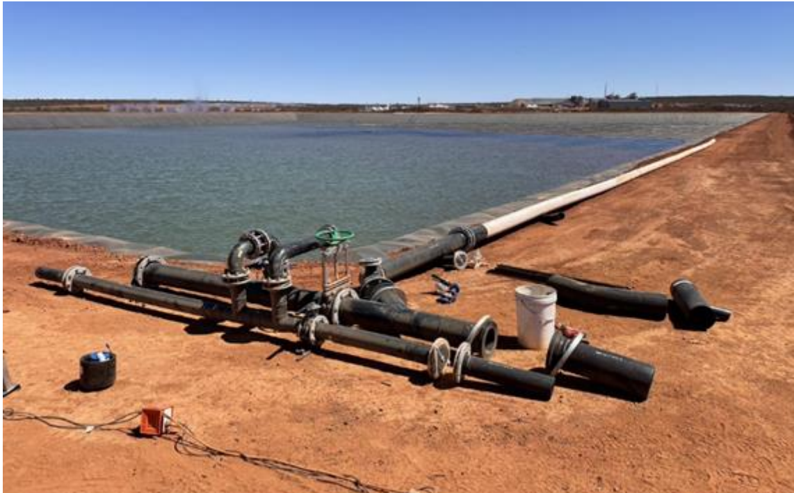
Figure 15 – TSF piping installation.
