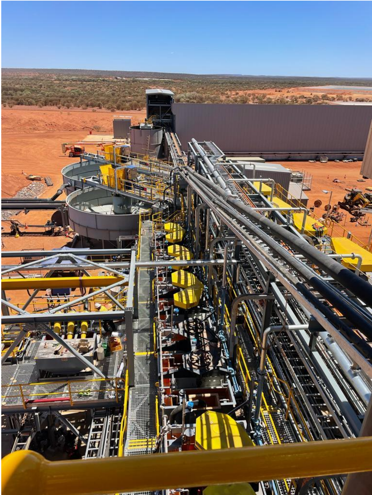
Figure 8 – Abra plant flotation, thickeners and concentrate shed with camp in the distance (Photo 11 November).
