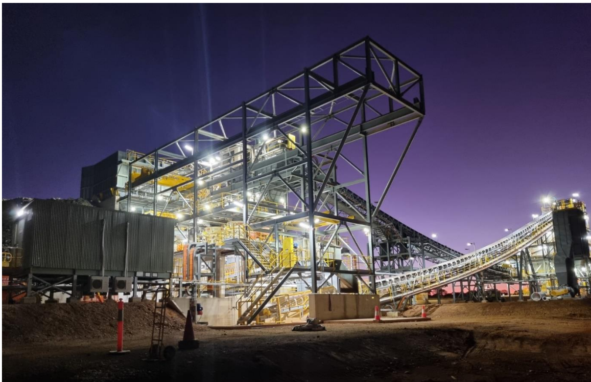
Figure 1 – Crushing and screening section energised for dry commissioning (Photo 9 November).
