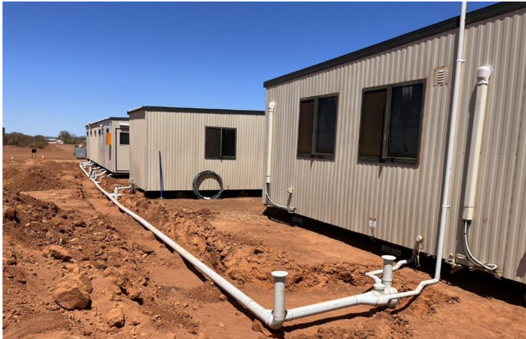
Figure 16 – Installation of processing plant buildings.
