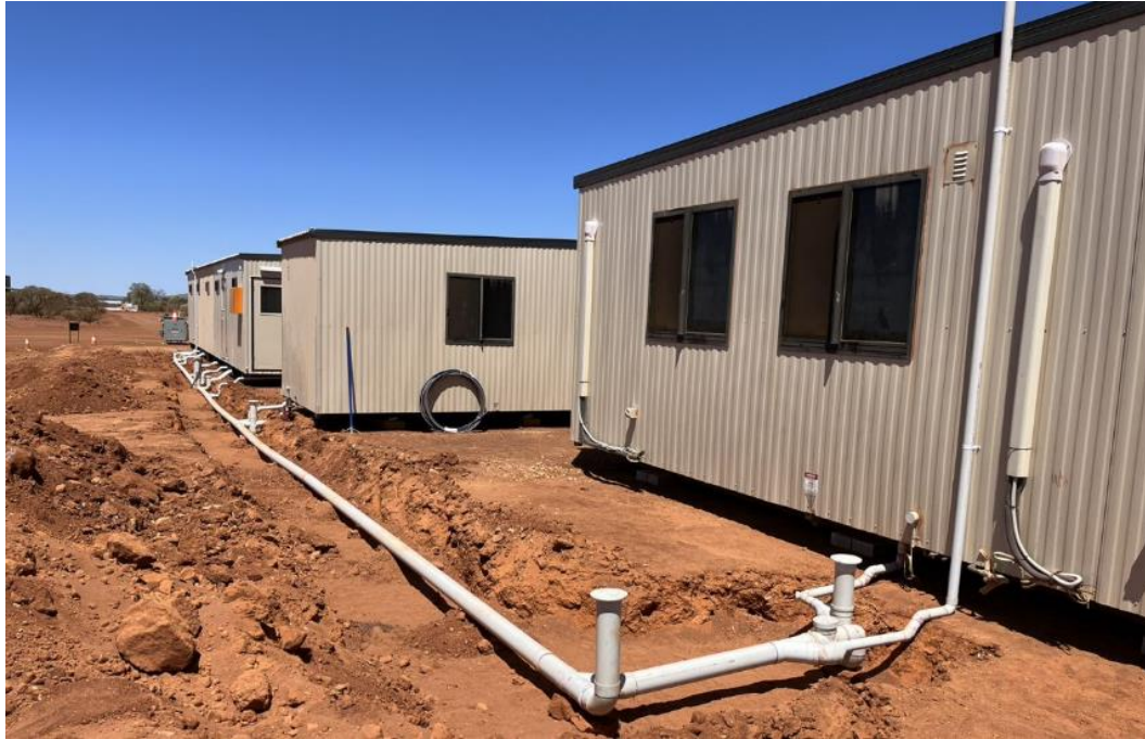
Figure 16 – Installation of processing plant buildings.
