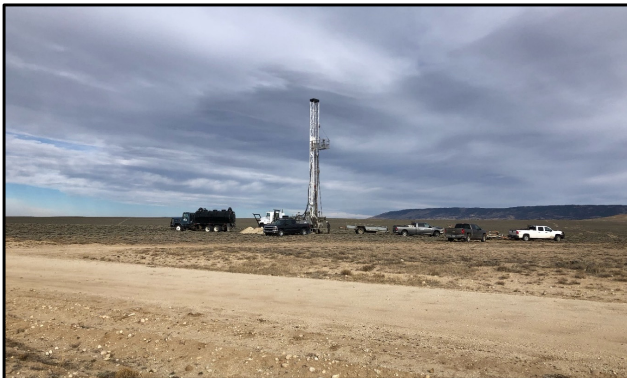
FIGURE 7. MUD ROTARY DRILL RIG OPERATING, ODIN ISR URANIUM PROSPECT, GDB WYOMING
