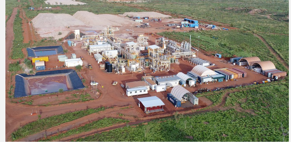
Northern Minerals Limited Browns Range Pilot Plant
