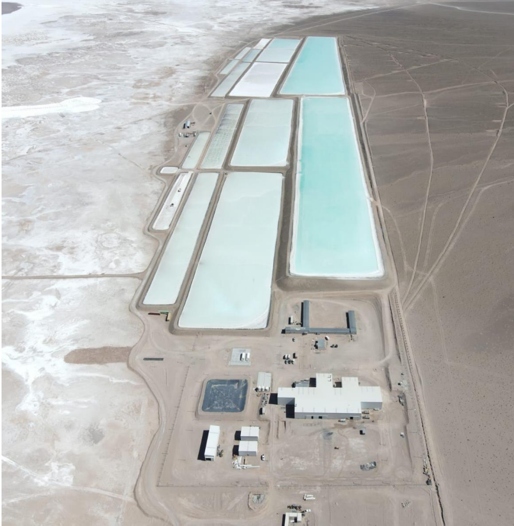
Figure 4. Rincon Lithium Project – 2,000tpa Operations Site
