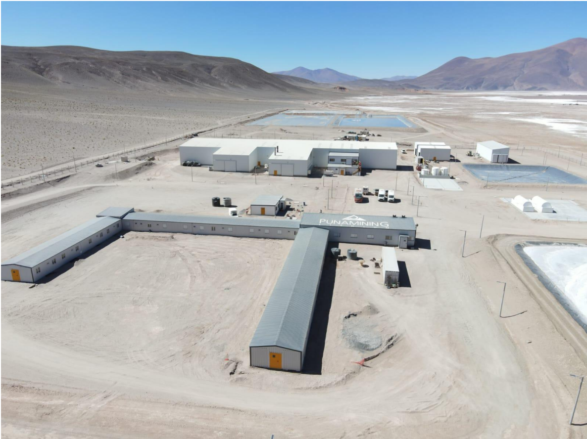
Figure 9. Rincon Lithium Project – 2,000tpa Operations Site
