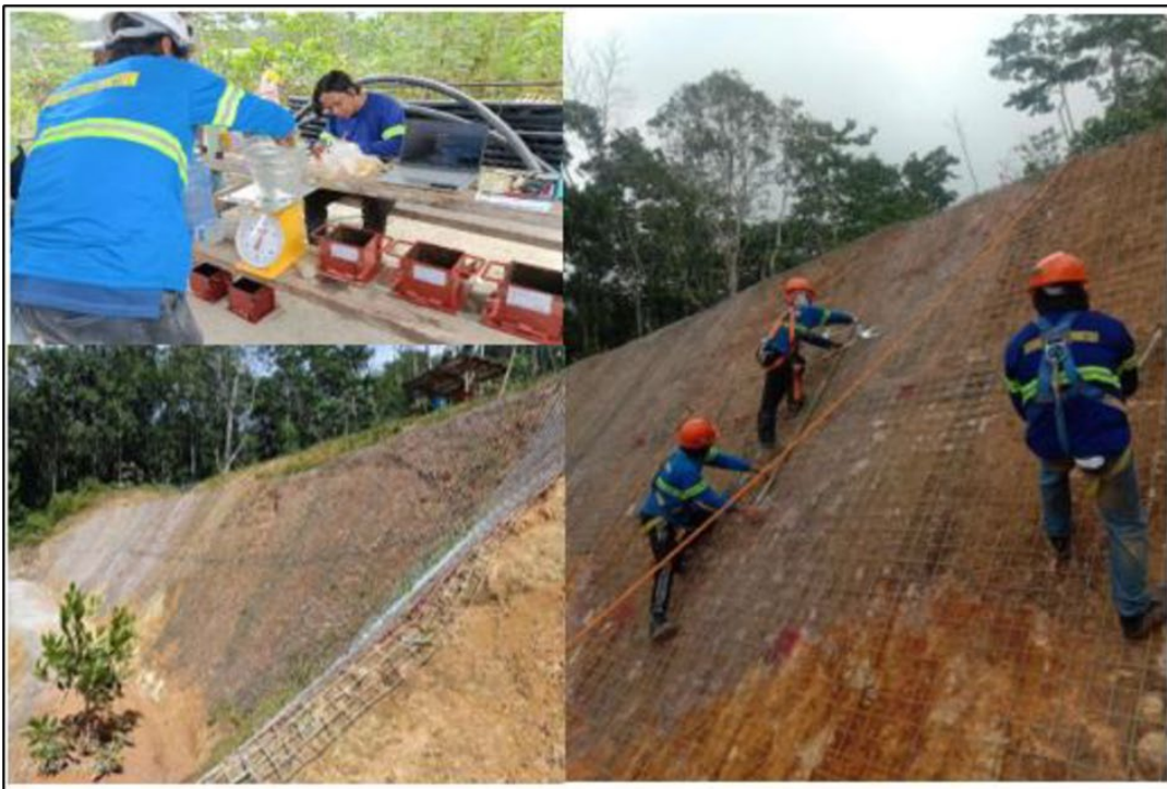
Photo 1: Wiremesh Installation at the Portal Slope
