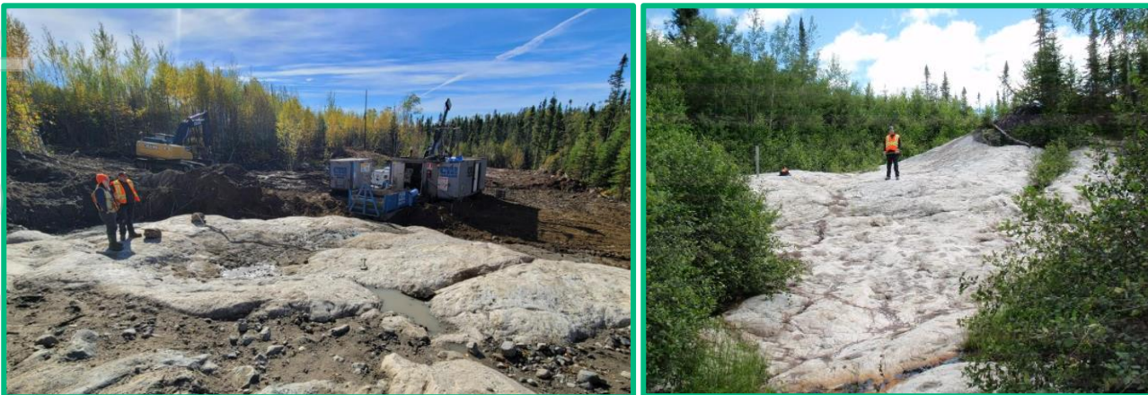
Figure 1: Drilling at the Seymour project
