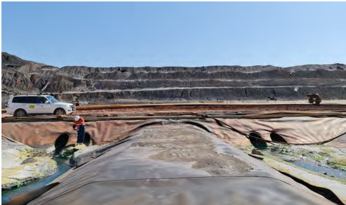
Image 4 / Leach Solution from Heap Drains – twin drains of copper sulphate solution
