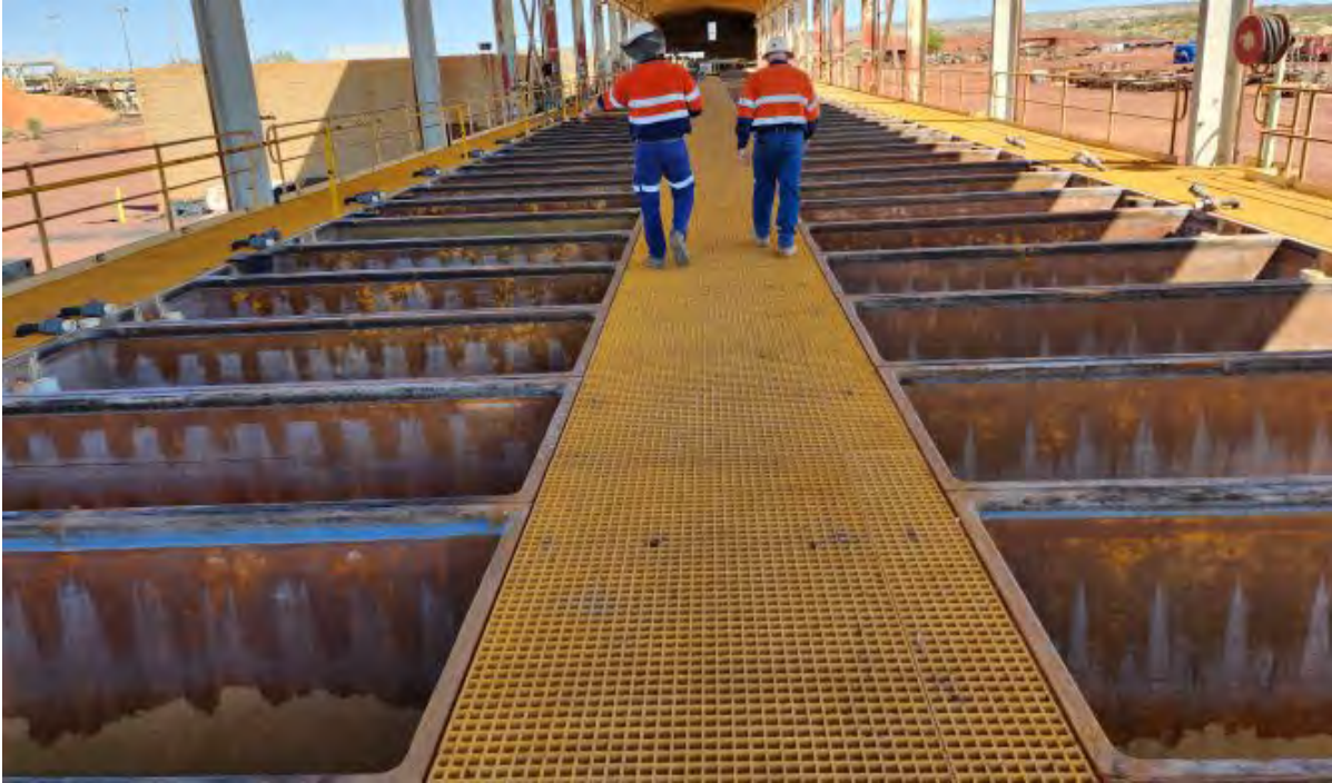
Image 8 / EW cells stripped of anodes and cathodes, cleaned and hydrotested waiting for refurbishment
