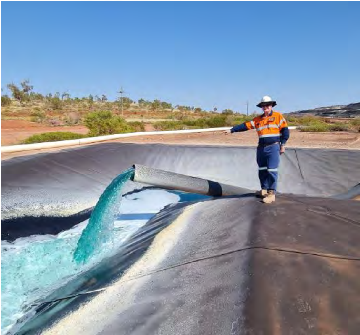
Image 5 / Leach Solution pumped from collection ponds to PLS pond – blue copper sulphate solution
