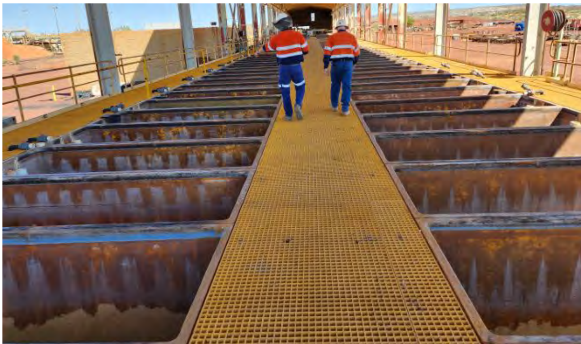
Image 8 / EW cells stripped of anodes and cathodes, cleaned and hydrotested waiting for refurbishment
