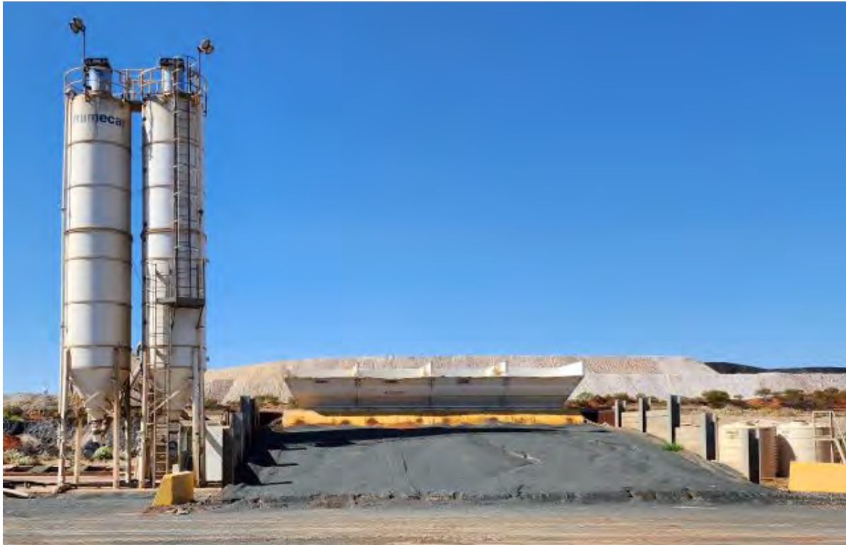
Image 12 / Concrete batching plant cleaned and serviced – ready to go
