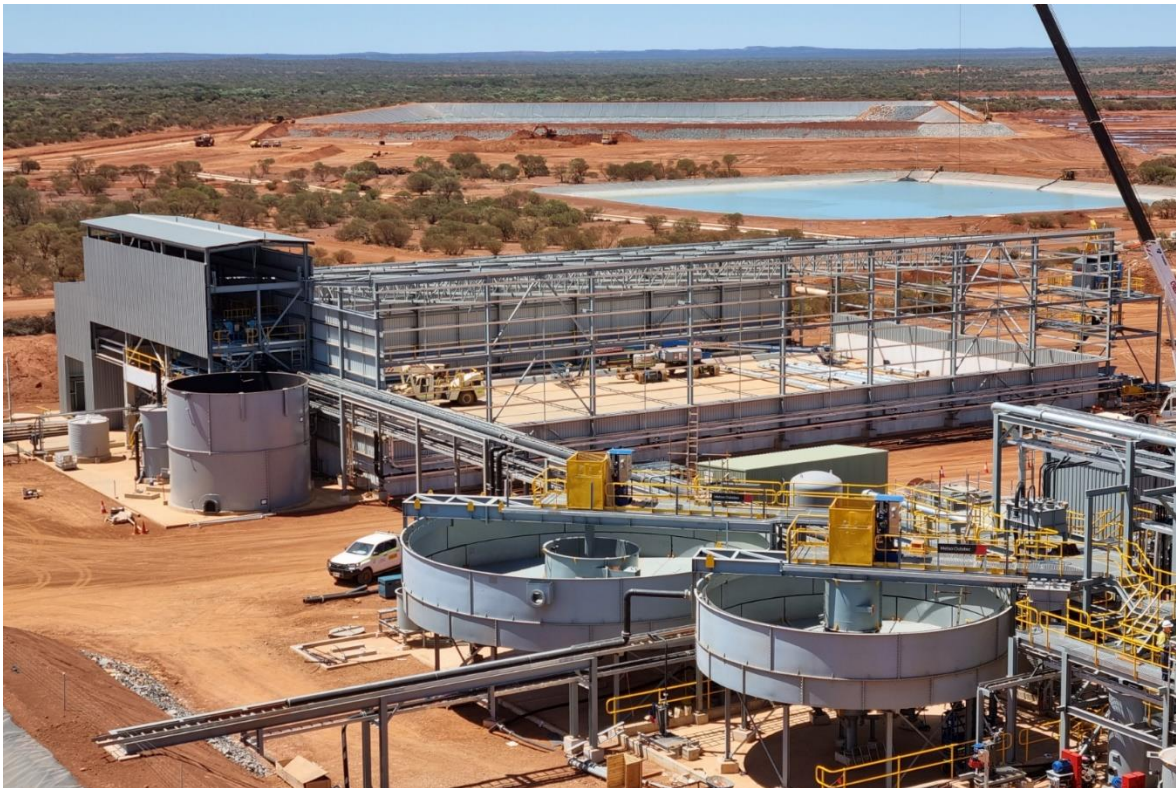
Figure 9. Processing plant concentrate section including thickeners and concentrate storage shed (Photo – 14 October 2022).
