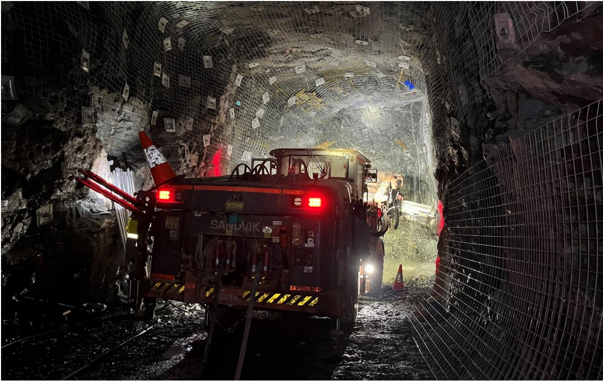
Figure 11. Abra underground decline development (Photo 30 September 2022).
