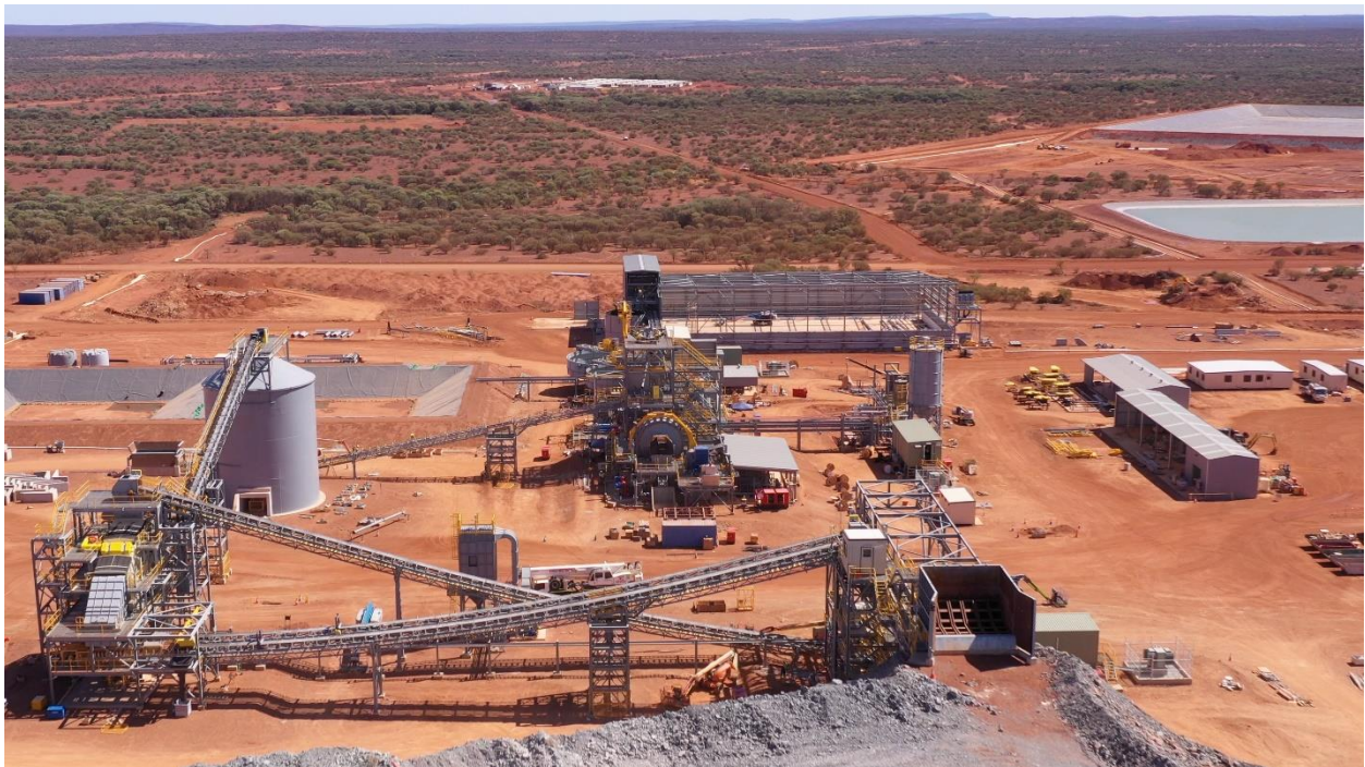
Figure 4. Abra processing plant progress in early October with TSF and village seen in the background (Photo – 14 October 2022).
