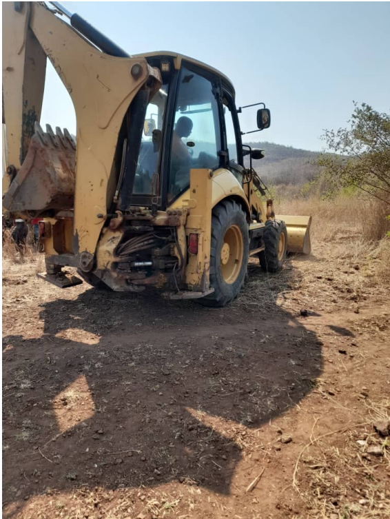
JCB onsite repairing hill top access roads
