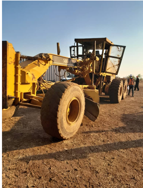
Grader on site maintaining access road
