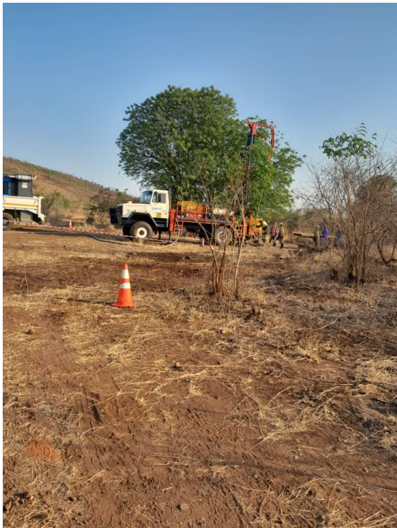
Drill rig and drill site
