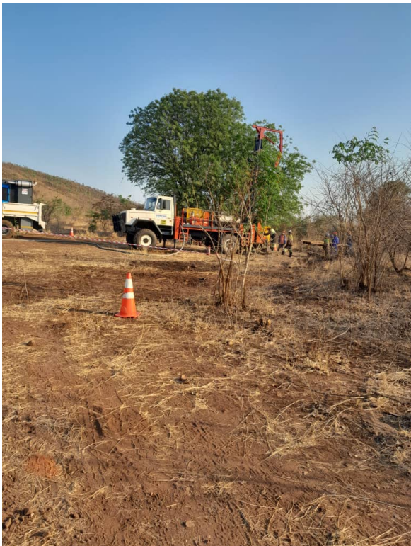
Drill rig and drill site
