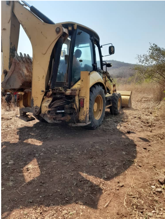
JCB onsite repairing hill top access roads
