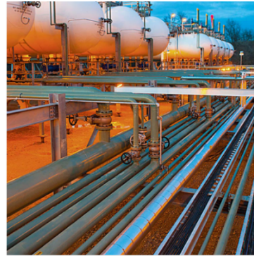
Most of the world's 3.5m kms of high pressure gas and oil pipelines contain niobium to make them safer, lighter and able to transport large volumes of hydrocarbons at higher pressures.
