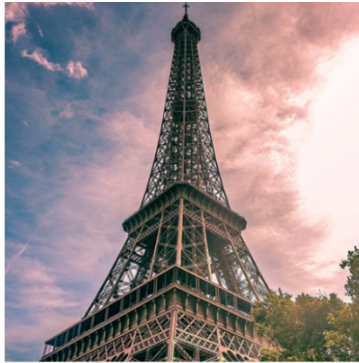
Construction of the Eiffel Tower in Paris used 7,300t of wrought iron. Today it could be built using only 2,000t of HSLA steel
