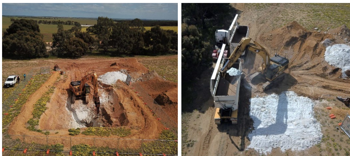
Figure 6: Test-pit in progress
