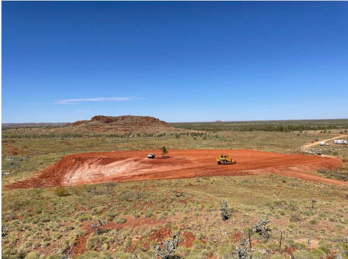
Figure 15. Exploration camp construction underway with levelling and compaction of 70m x 70m area in preparation for dome-sheltered core yard, accommodation, ablution block, workshop and offices. The prominent hill in the background is the part of the Main Hill prospect. View looking south.
