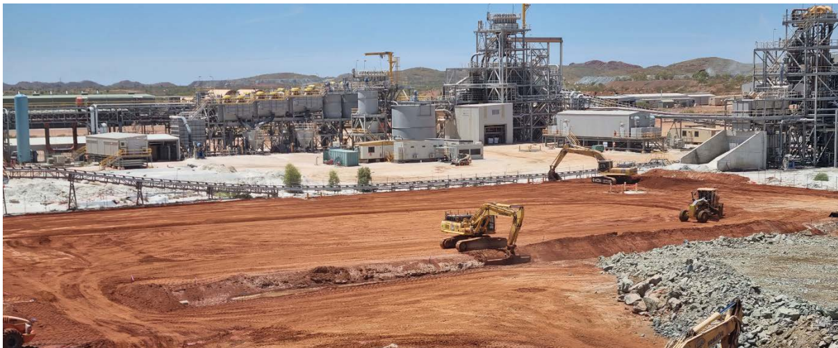
Figure 2: Bulk earthworks underway for P680 project
