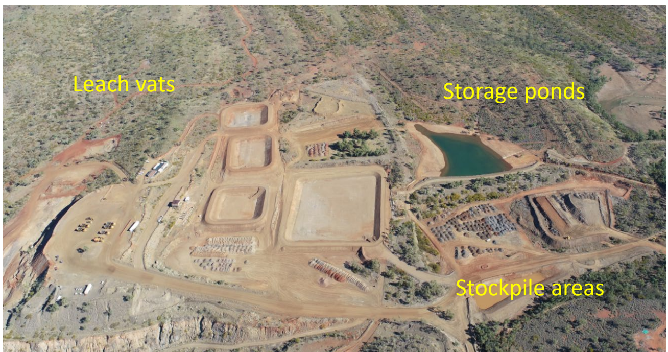
Image 6 - Mt Freda Complex - showing leach vats, storage ponds and stockpile areas.
