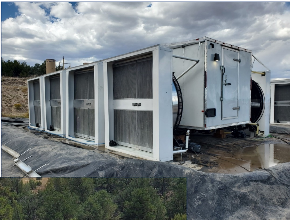
Figure 1 Cooling Modules Installed at Elite Mobile Unit
