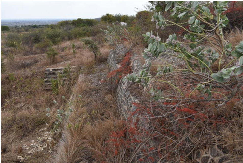
Figure 6: Retaining wall of historic pilot plant crusher
