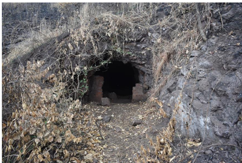
Figure 5: Entrance to historic adit
