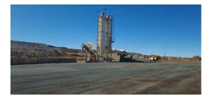
A concrete batch plant was commissioned in early 2018. The plant is capable of 80m³ of general use concrete per hour. The plant will be used in the operational restart and construction phase for the concrete demand from these activities.
