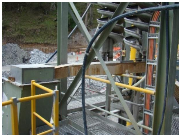
Figure 5 Hill End gold is highly amenable to gravity recovery
