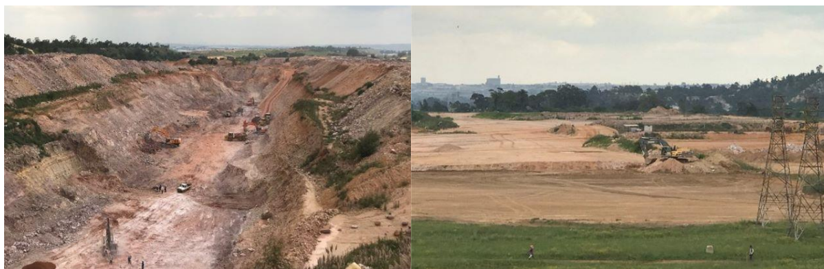
IMAGE 12: QALA SHALLOWS OPEN-PIT MINE BEFORE (LEFT) AND AFTER (RIGHT) REHABILITATION
