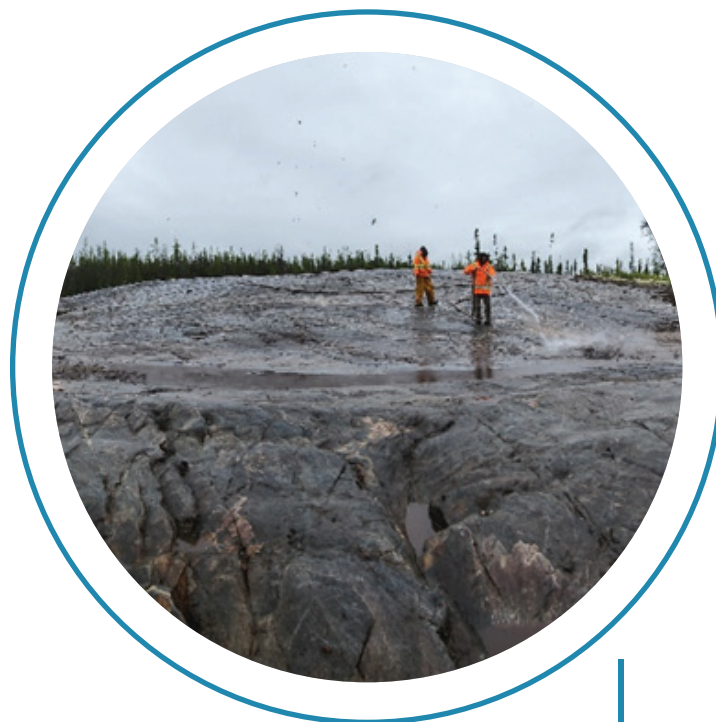
Preliminary stripping of vegetation to expose Cancet main dyke
