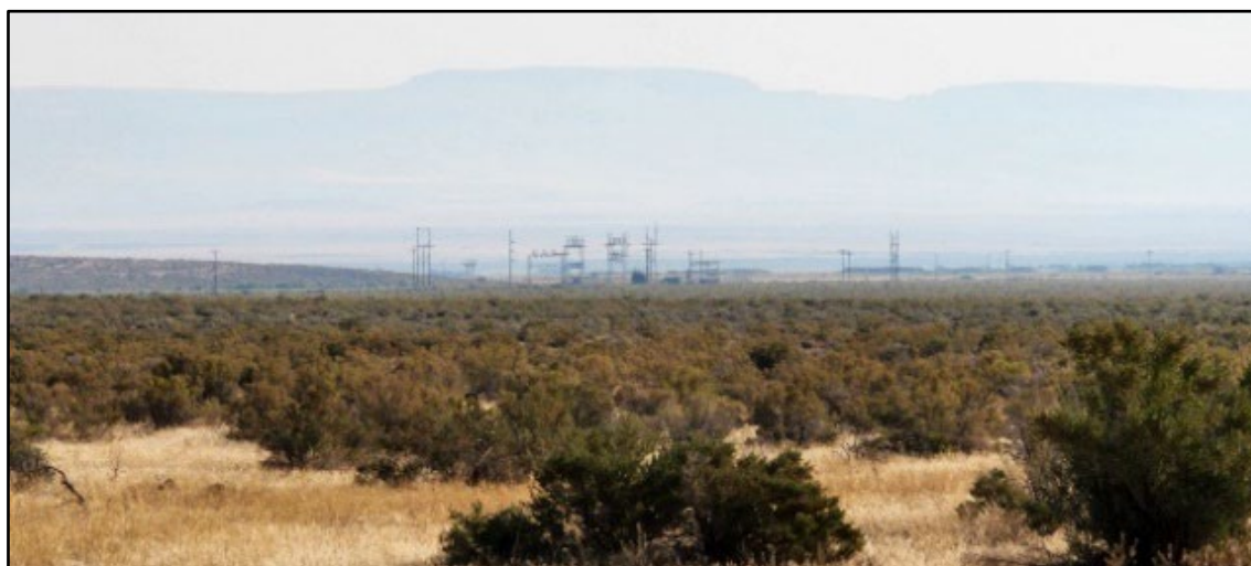
Figure 3: View across acquired land to substation
