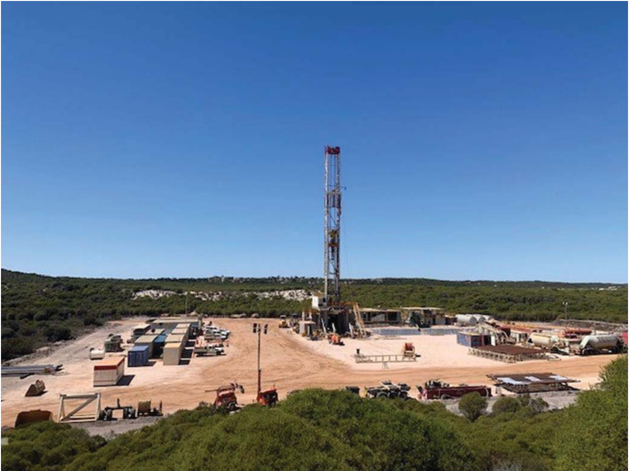
Figure 3: Ensign 970 drilling at Cervantes-1 location
