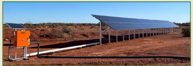
Borefield powered by a solar array.
