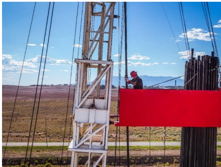
Figure 4: Work-over Rig on Jesse#1A with the Abajo mountains in the background
