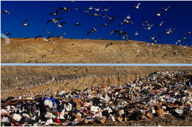
The blue highlighted line indicates where a manufactured zeolite layer could function to intercept and oxidise methane emitted from the underlying refuse
